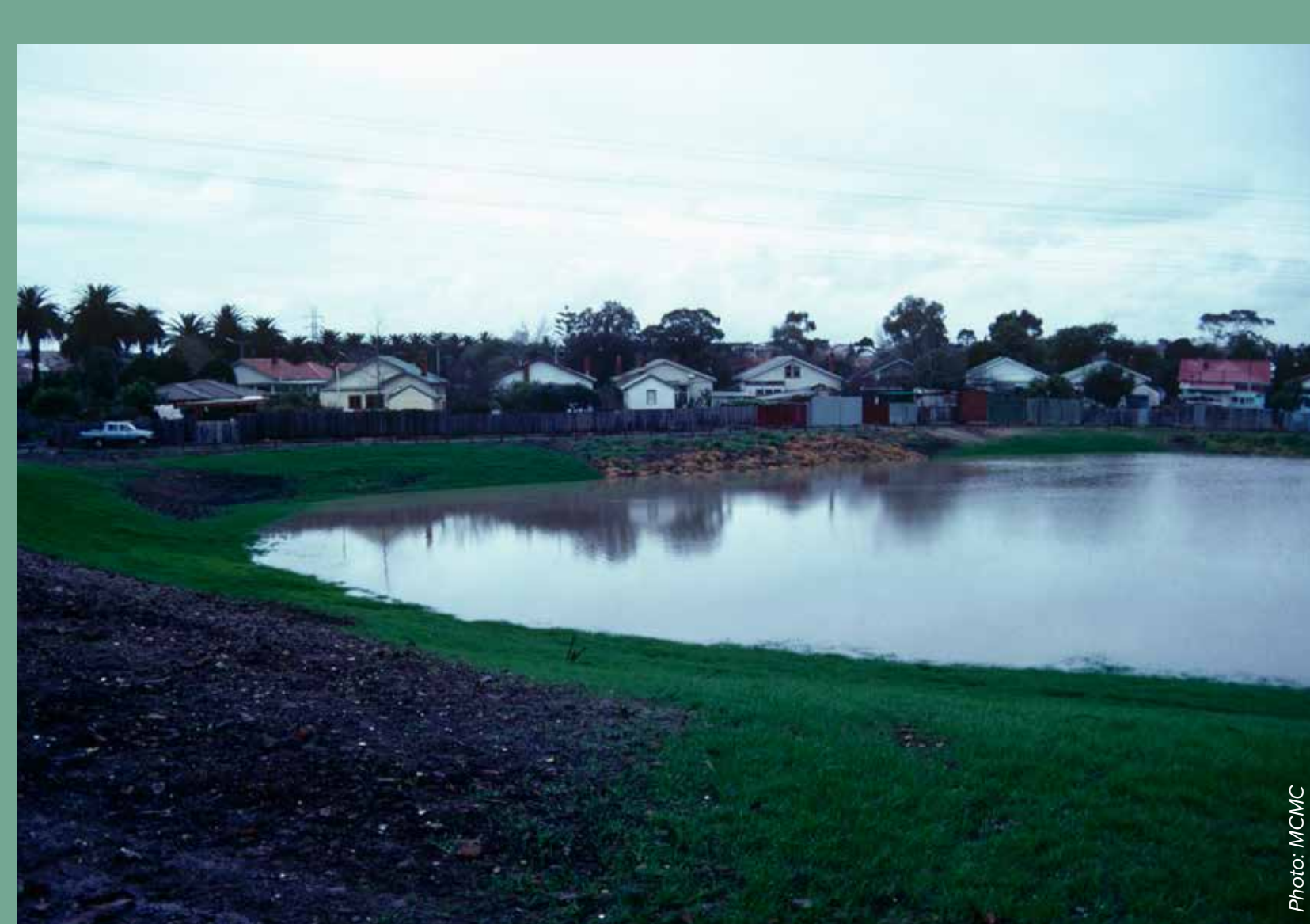
Before: The Merri Park retarding basin in flood in 1990.
